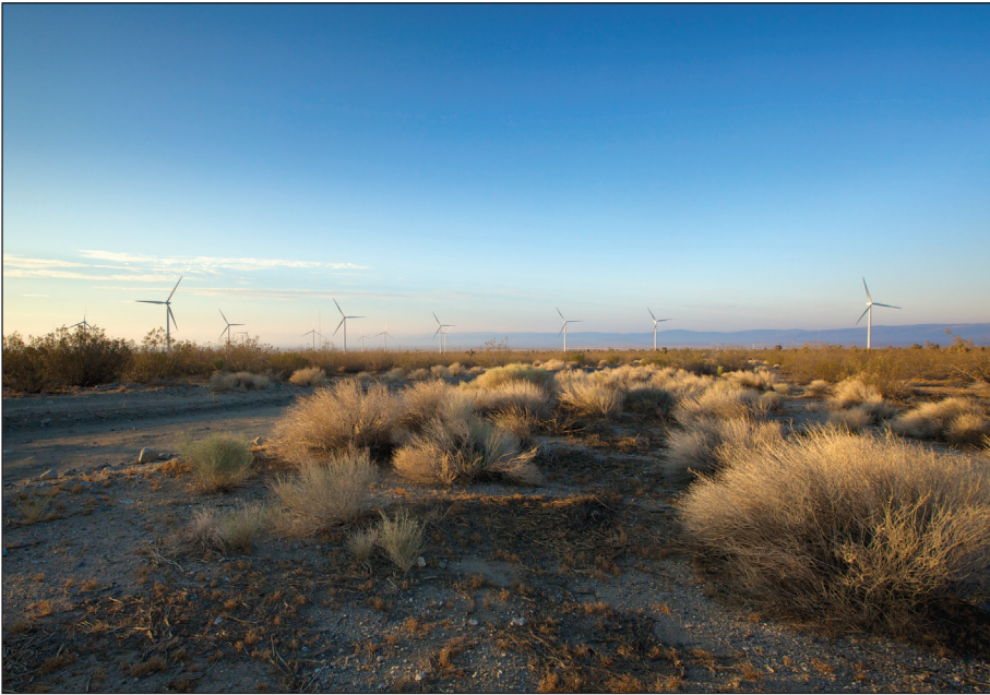
A panoramic shot of EDF Renewable Energy's 140 MW Pacific Wind Farm.
